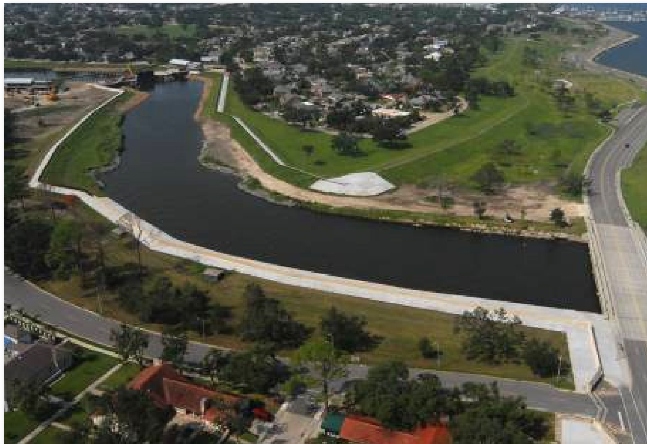
Flood protection improvements such as armored floodwalls are key to recovery throughout all of New Orleans.
